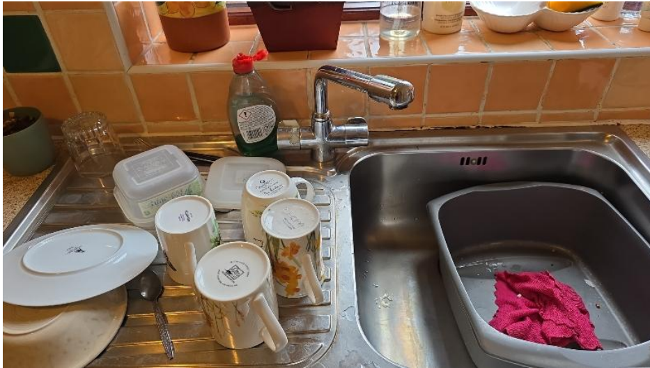
Sealant and repairs required to kitchen worktop
