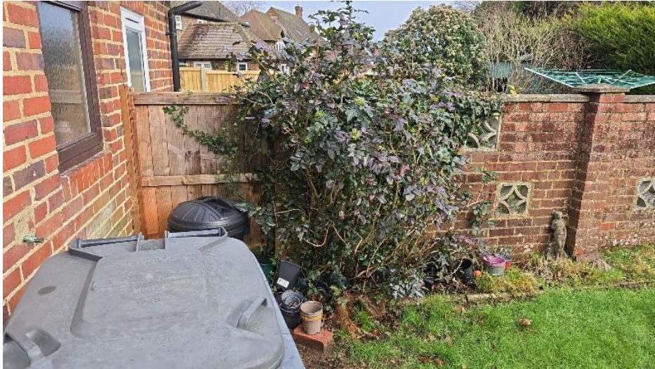
Vegetation restricting our inspection
