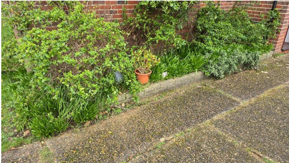
Raised plant beds close to DPC level
