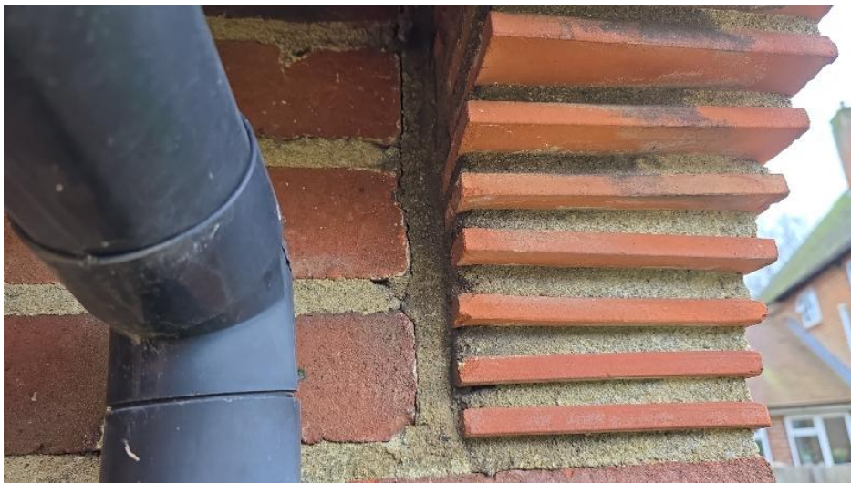
Vertical cracking
