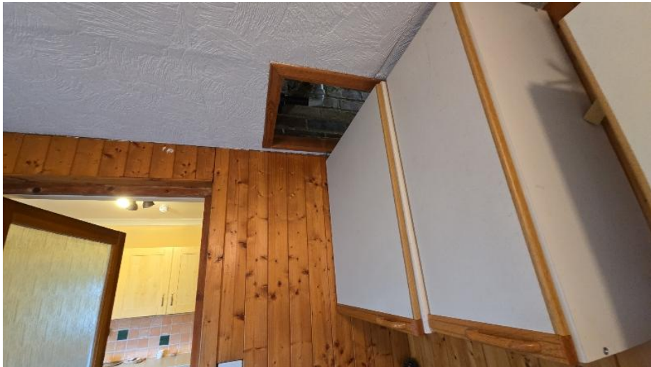
Partially concealed loft access to utility room
