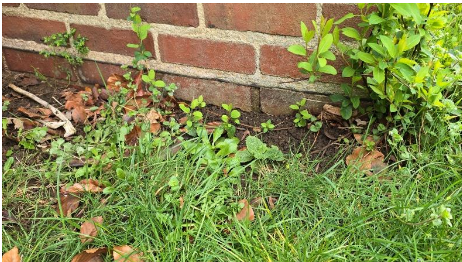
Raised plant beds close to DPC level
