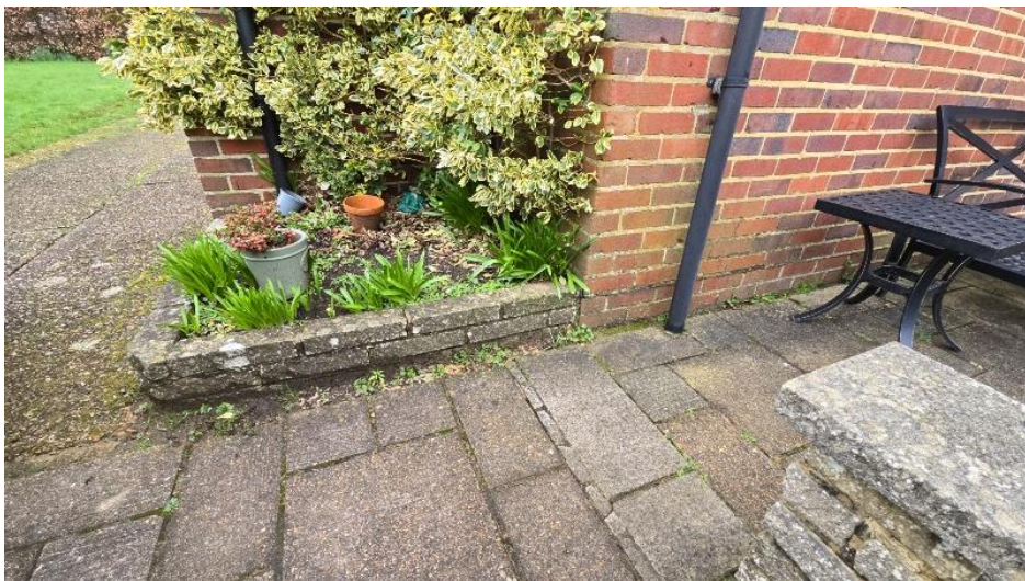
Raised plant beds close to DPC level
