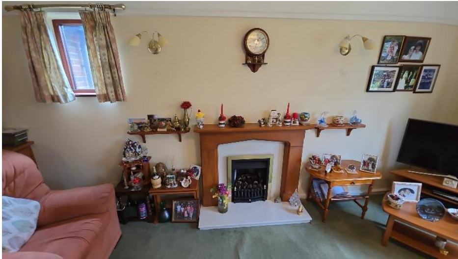
Gas fire to living room, external chimney stack
