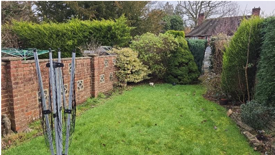
Vegetation restricting our inspection
