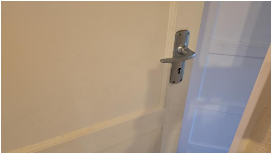
Doors general ironmongery repairs or replacement throughout
