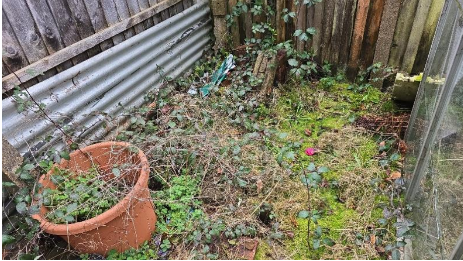
Vegetation growth limiting inspection
