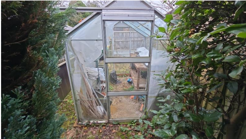
Existing greenhouse inspect for safety glazing markings
