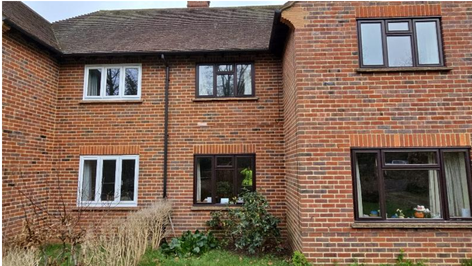
Shared rainwater goods with neighbouring property
