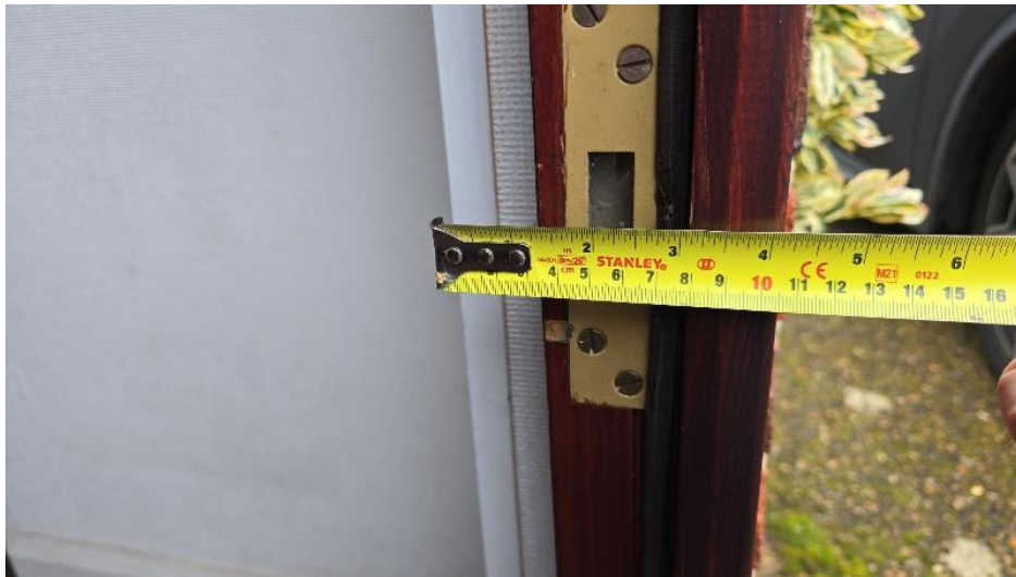
Single brick thick Porch wall with fibre board lining internally
