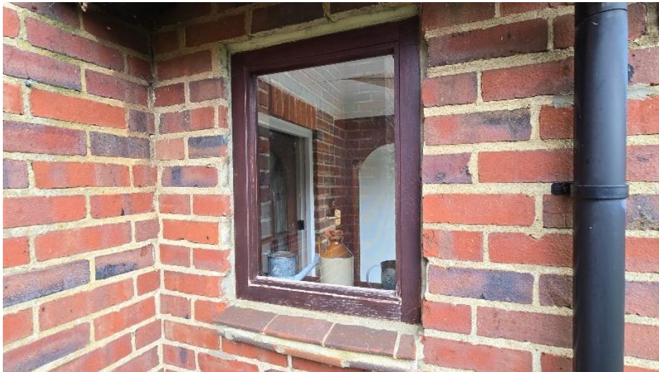
Single glazed porch window
